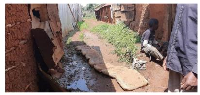
Figure 19: Used cement bags filled with soil to control runoff.
