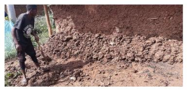
Figure 18: Heaping mud on shack base for stability.
