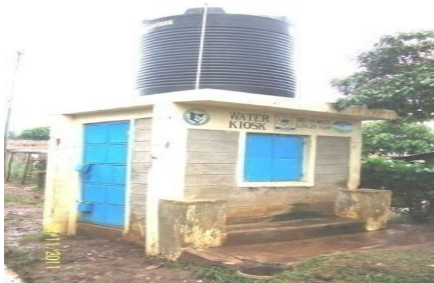
Plate V: Municipal Water Kiosk at Kisumu Ndogo (Source: Author, 2011)
