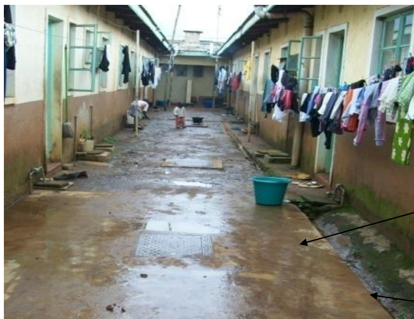
Wet concrete yard
