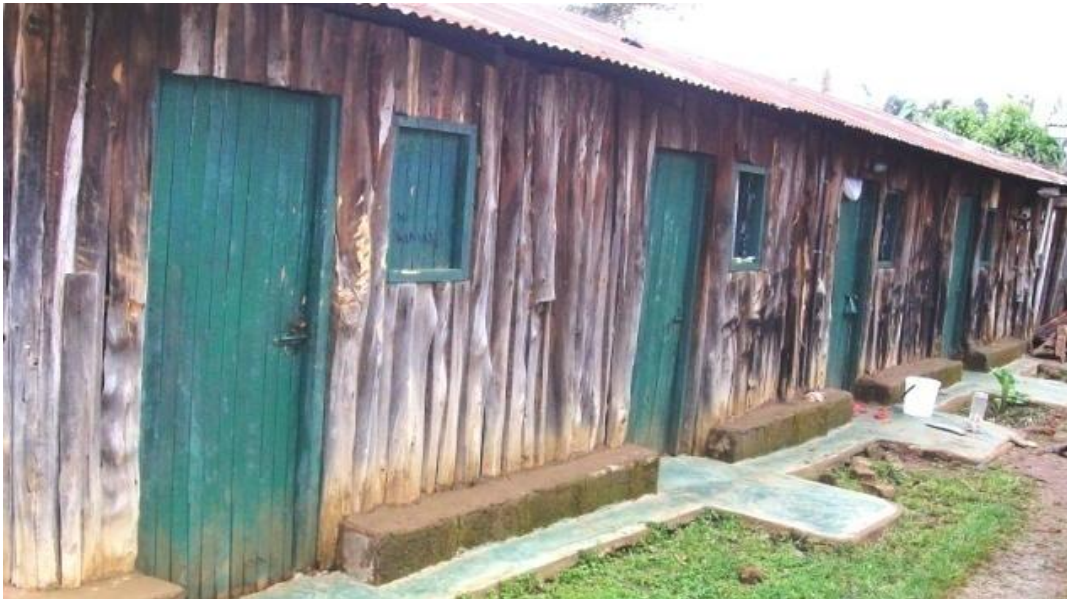
Plate AD: Woodwall, cement floor house at Kasarani
