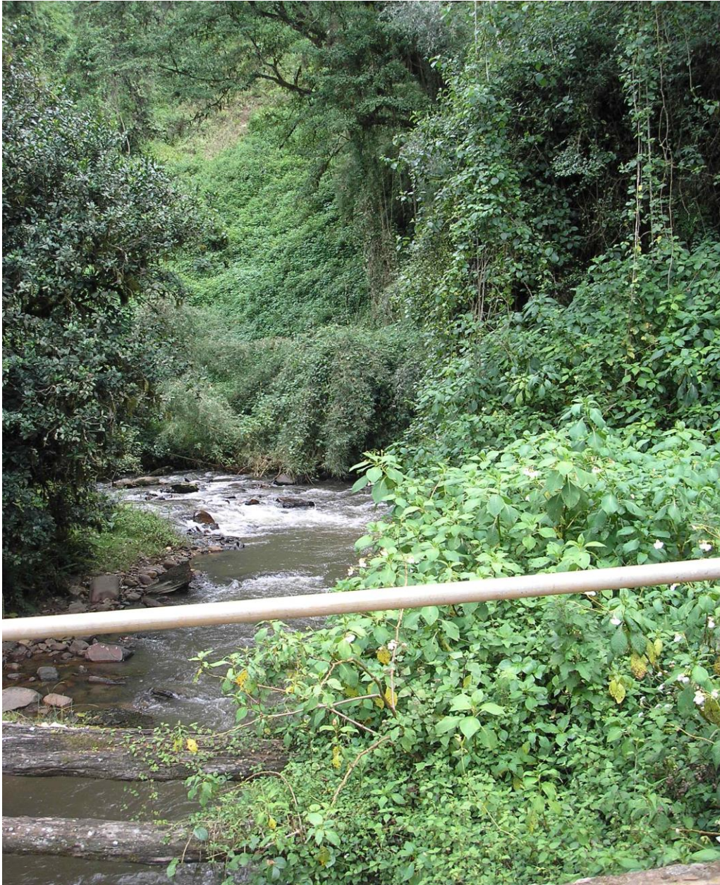
Plate 4.1: One of the pipe that was used to supply water to the farms located downstream
