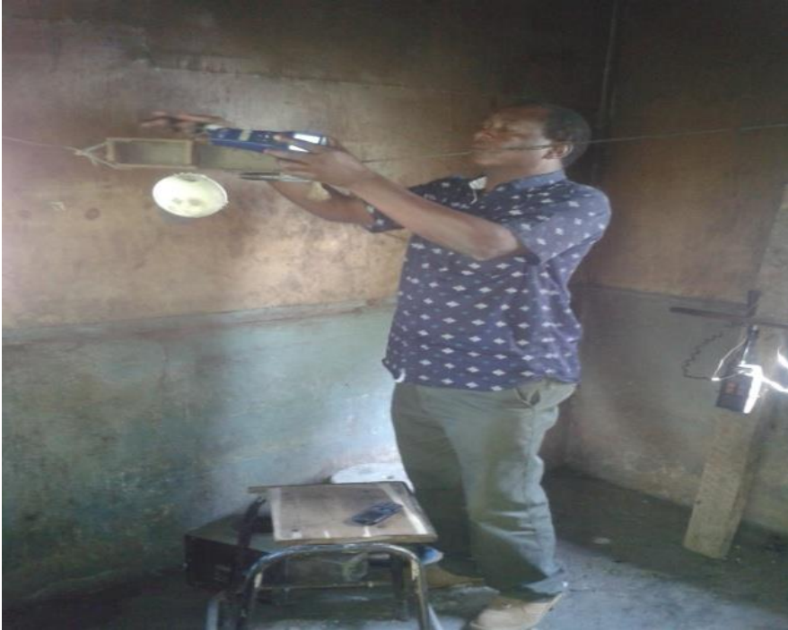
Appendix G 8: Mounting Emission gas meters (Source: Author, 2016)
