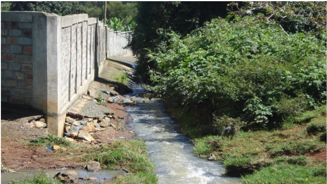
Plate 6: Monopitch Housing development type encroaching on natural water drain in Elgon View Low Density Neighbourhood. Source: Field Data
